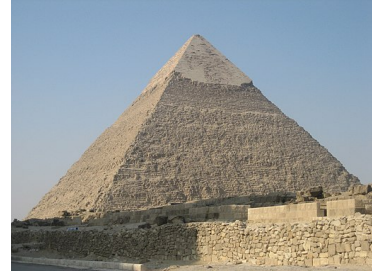
Khafre's pyramid at Giza. At the top of the pyramid you can see many remaining casing stones. Image by Daaaveee, commons.wikimedia.org
